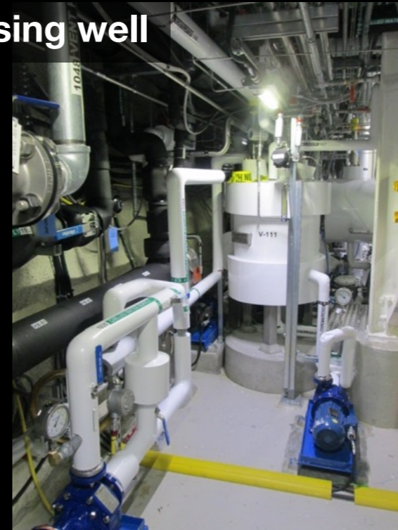
Tellurium purification and loading systems completed: undergoing commissioning
